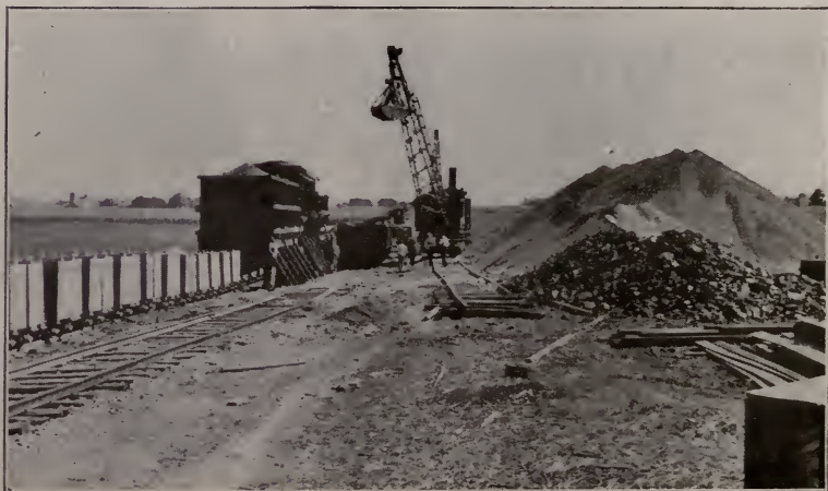
Fig. 8. Material plant for central proportioning batch boxes for industrial railroad delivery.
