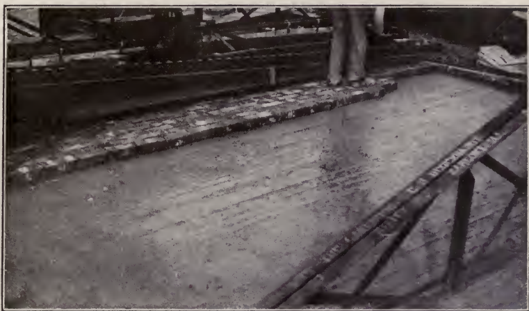
Fig. 20. Monolithic brick road showing concrete base and brick surface being finished with a mechanical tamping and finishing machine.
