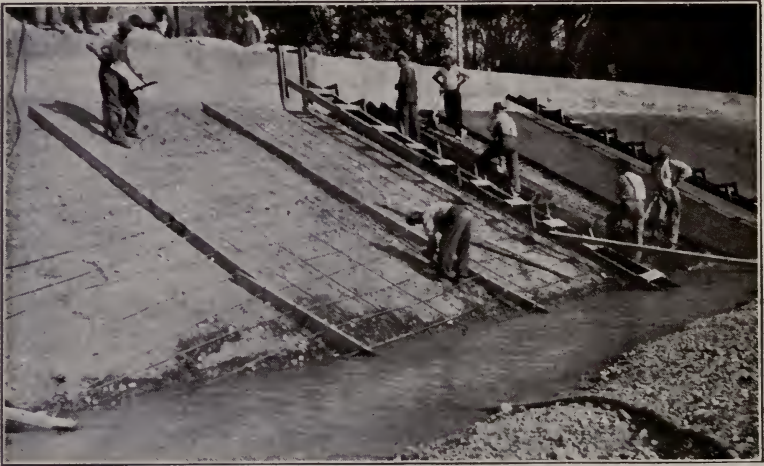
Fig. 14. Slope-wall construction to protect road from excessive erosion.
