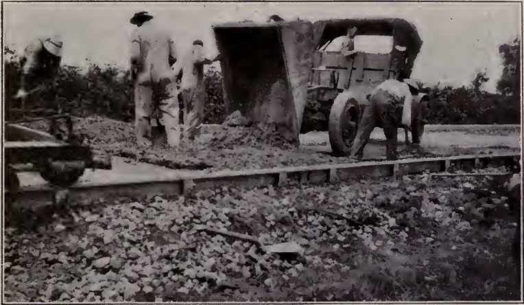
Fig. 5. One and one-half ton pneumatic tired truck delivering mixed concrete from central plant to road.
