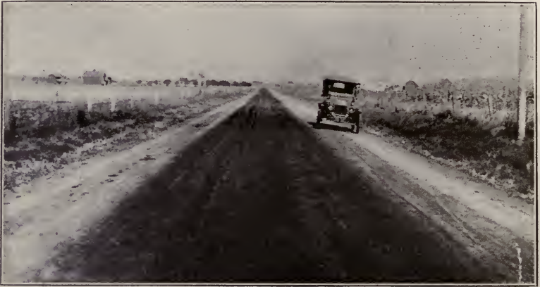
Fig. 27. Well graded and oiled earth road.
