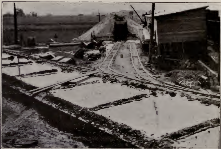
Fig. 7. Concrete pavement cured by ponding method. Note tunnel and material yard and cement storage bins in background.
