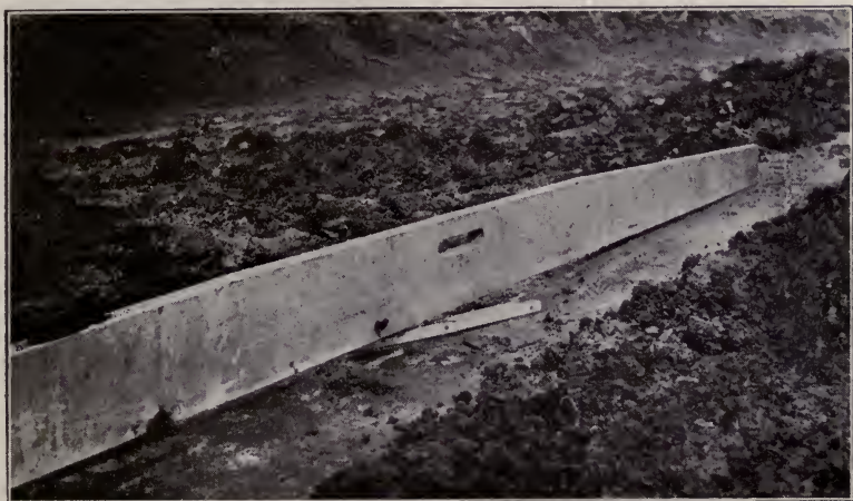
Fig. 13. Ten-foot straight edge shows up a depression of three-fourths inch in the finished surface.
