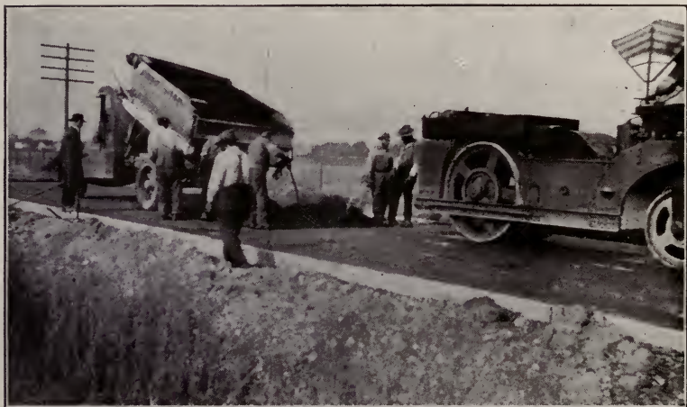
Fig. 22. Dumping, spreading, and rolling bituminous concrete on a concrete base.
