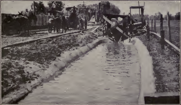
Fig. 1. Temporary reservoir adjacent to deep well to hold surplus water during paving operations.
