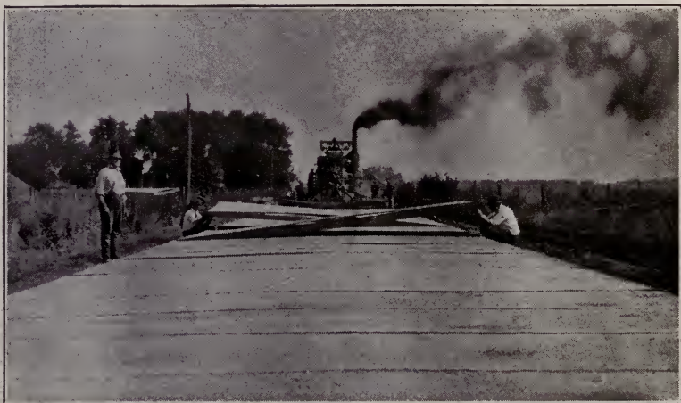
Fig. 19. Canvas covered frames used to cover a concrete road immediately behind the paving mixer.
