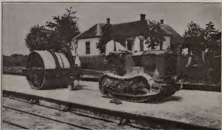
Fig. 3. Horse roller coupled to caterpillar tractor and used for rolling subgrade.
