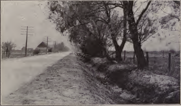
Fig. 28. Showing well shaped shoulder and side ditch.
