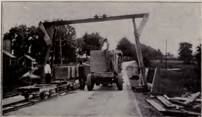
Fig. 9. Transfer station for material boxes from trucks to industrial cars. Industrial cars deliver materials to paving mixer about one mile ahead.
