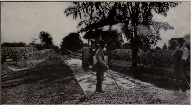
Fig. 23. Trench method of constructing macadam or gravel roads.
