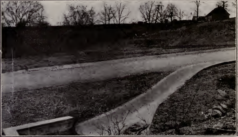
Fig. 16. Gutter section on steep grade and through a heavy cut.
