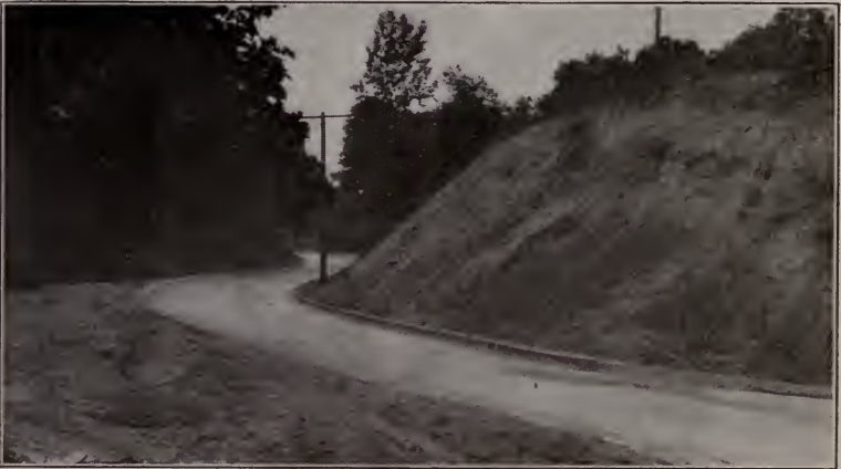
Fig. 17. Curb and gutter construction on steep grades and through heavy cuts.
