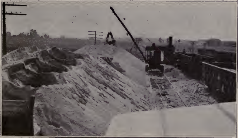
Fig. 6. Aggregate stored on top of a tunnel permits large storage of material and easy method of filling batch boxes on industrial railroad equipment.
