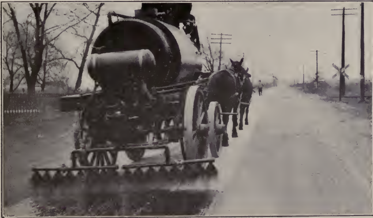
Fig. 25. Method used for distributing bituminous material for surface treatment of macadam and gravel roads or for oiling earth roads.
