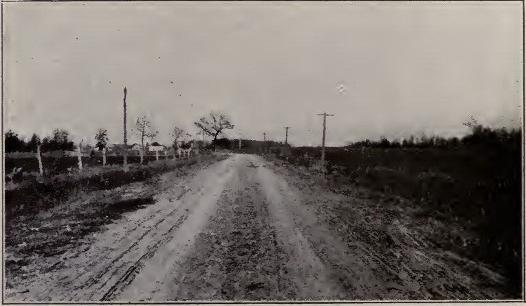
Fig. 24. Gravel road constructed by the feather-edge method.
