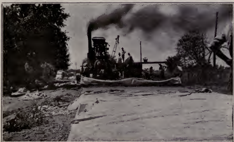
Fig. 18. Canvas covering on newly laid concrete pavement to protect it from sun and wind. Canvas should be kept wet when weather is extremely hot.
