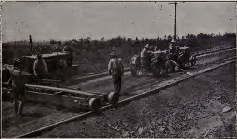
Fig. 2. Preparing subgrade in advance of a paving mixer.
