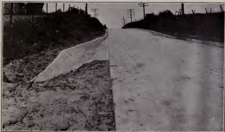
Fig. 15. Curb and gutter outlet at bottom of steep grade.
