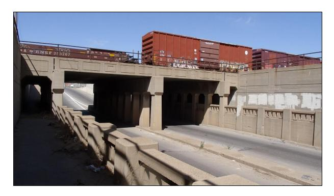
With the construction of the interstate system and further refinement of freeway design, grade-separation structures were commonly reinforced concrete girders, steel I-beams, steel girders, and (after the early 1960s) prestressed concrete girders. In 1960, the vertical clearance requirement over roadways was increased to 16 feet.<sup>13</sup>
