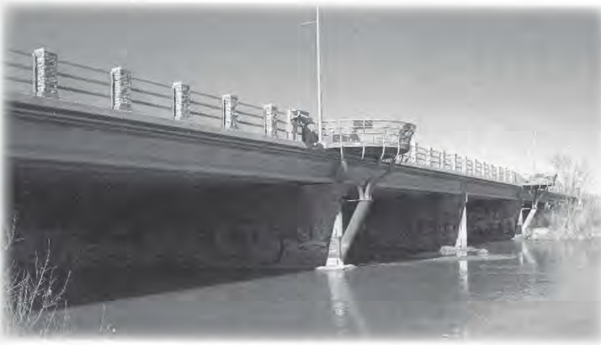
The current Central Avenue Bridge sits between levees and drainage ditches, as originally configured in 1930, and was integrated into the MRGCD flood control system. Three of the 16 spans are devoted to main channel flow, and the other spans are held in reserve for heavy flooding. (Norman Falk photo)
