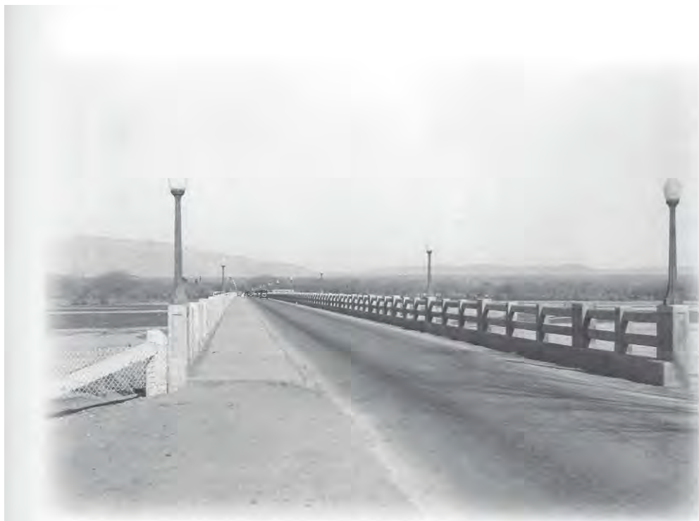
The Central Avenue Bridge was completed in 1930. (Courtesy Albuquerque Museum, Alabama Milner photographer, museum purchase)
