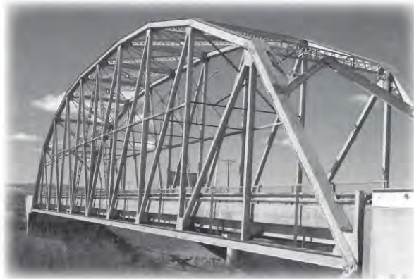
The Rio Puerco Bridge, completed in 1934, is one of a few Parker through-truss bridges left in the state. (Sherry Robinson photo)
