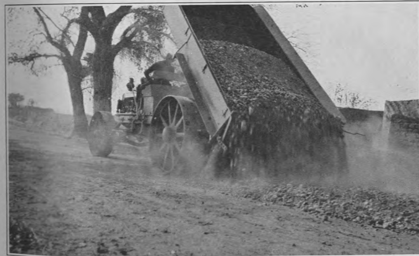
VALENCIA COUNTY. State Road truck spreading gravel on Road 1. Sec. 1.
