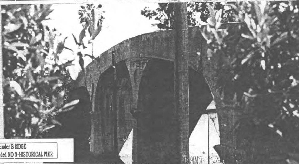
View North of BRIDGE span #2 detail of added NO N-HISTORICAL PIER
