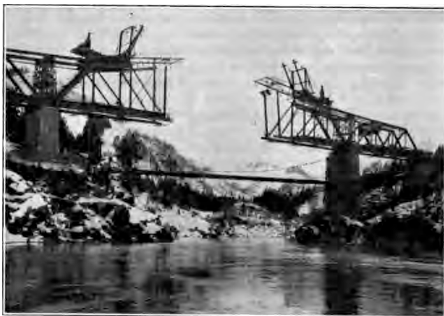
FIG. 25e. Simple-truss Bridge on the Nippon Railway in Japan, Erected by the Cantilever Method.
