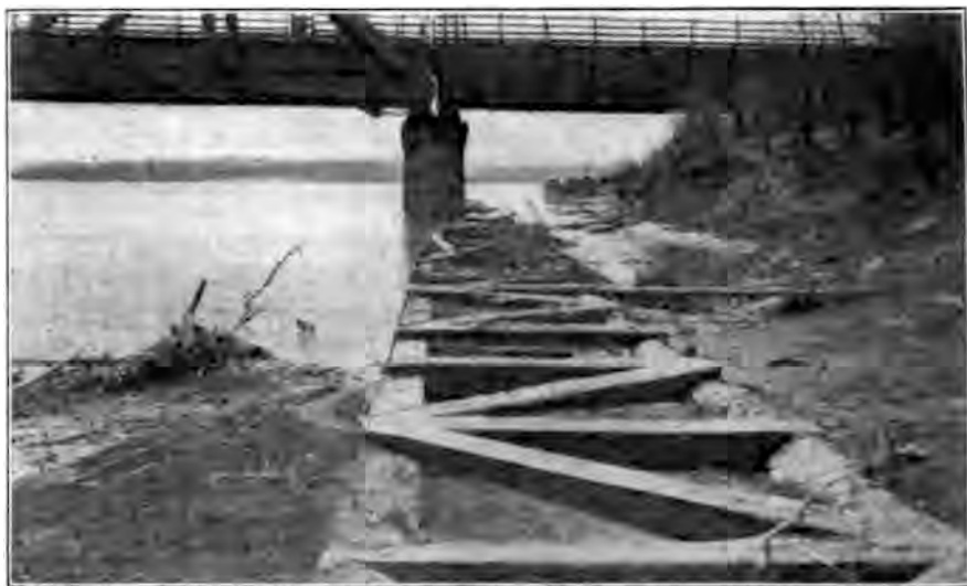
FIG. 44a. Shore Protection on the Nebraska Side of the Missouri River at East Omaha, Neb.
