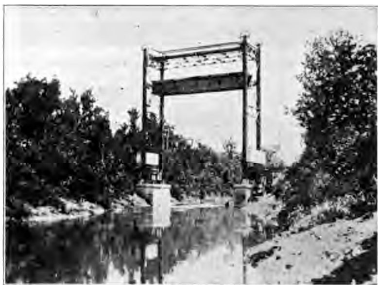
FIG. 31i. Vertical Lift Bridge over the Big Choctaw Bayou, Louisiana, on the Line of the M. L. and T. R. R. & S. S. Co.—Span Up.
