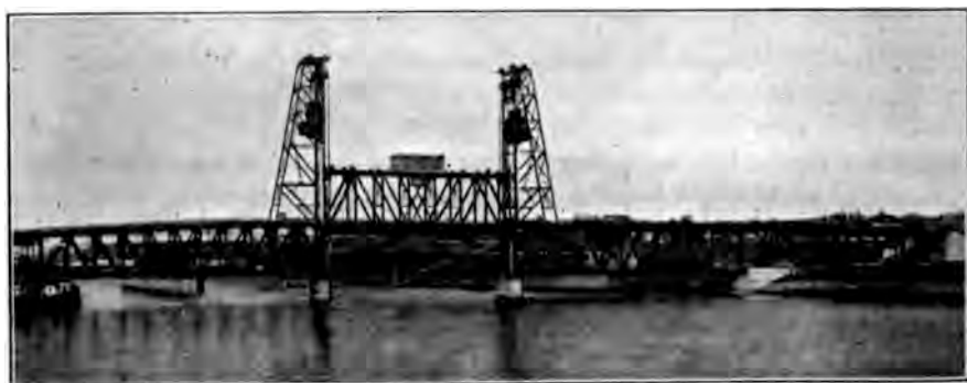
FIG. 31k. O.-W. R. R. and N. Co.'s Bridge over the Willamette River at Portland, Ore.—Lifting Deck Up.
