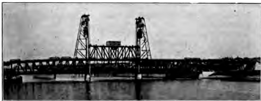
FIG. 31j. O.-W. R. R. and N. Co.'s Bridge over the Willamette River at Portland, Ore.—Lifting Deck and Lifting Span Down.
