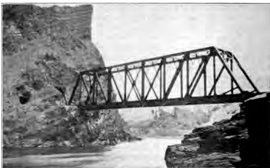
FIG. 25h. Simple-truss Bridge over the Thompson River on the Line of the Canadian Northern Pacific Railway in British Columbia, Erected by the Cantilever Method.
