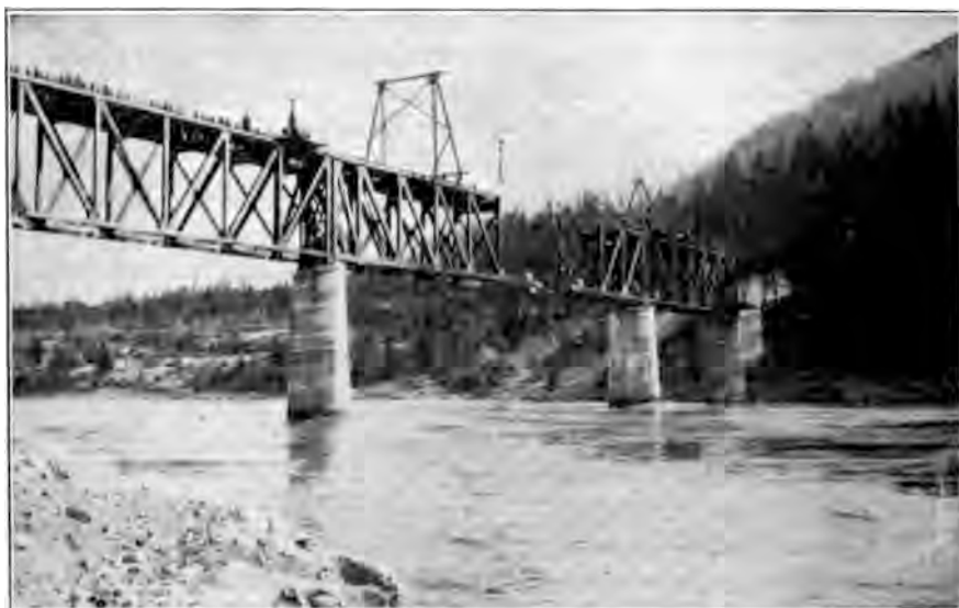
FIG. 25g. Simple-truss Bridge over the Fraser River on the Line of the Canadian Northern Pacific Railway in British Columbia, Erected by the Cantilever Method.
