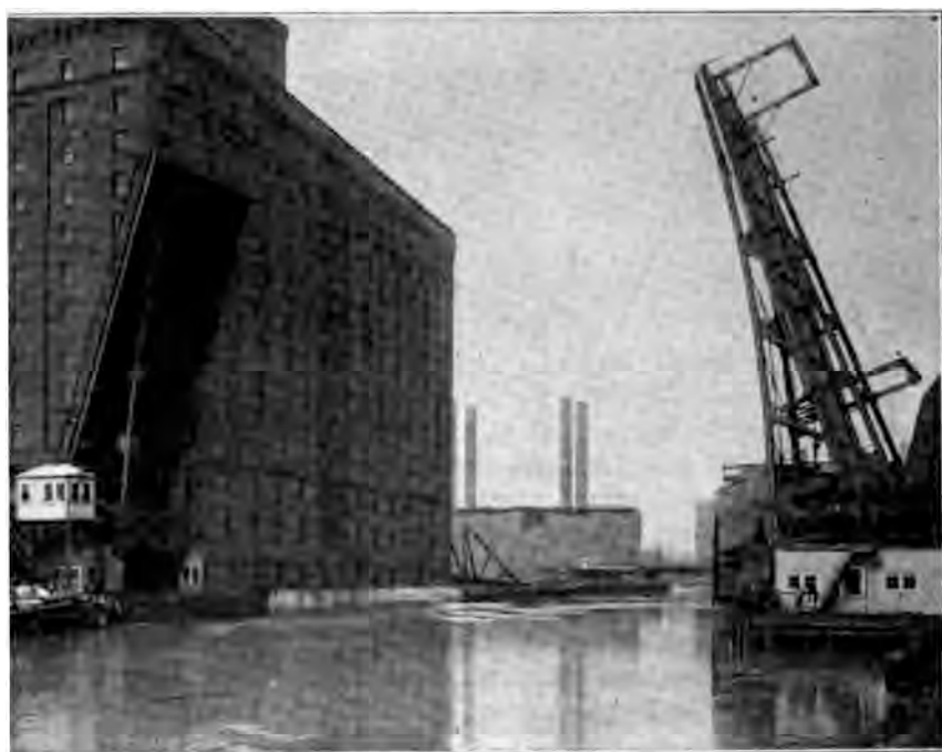
FIG. 30f. Strauss Bascule Bridge at Polk Street, Chicago, Ill.
