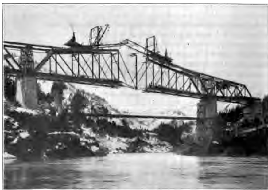
FIG. 25f. Simple-truss Bridge on the Nippon Railway in Japan, Erected by the Cantilever Method.
