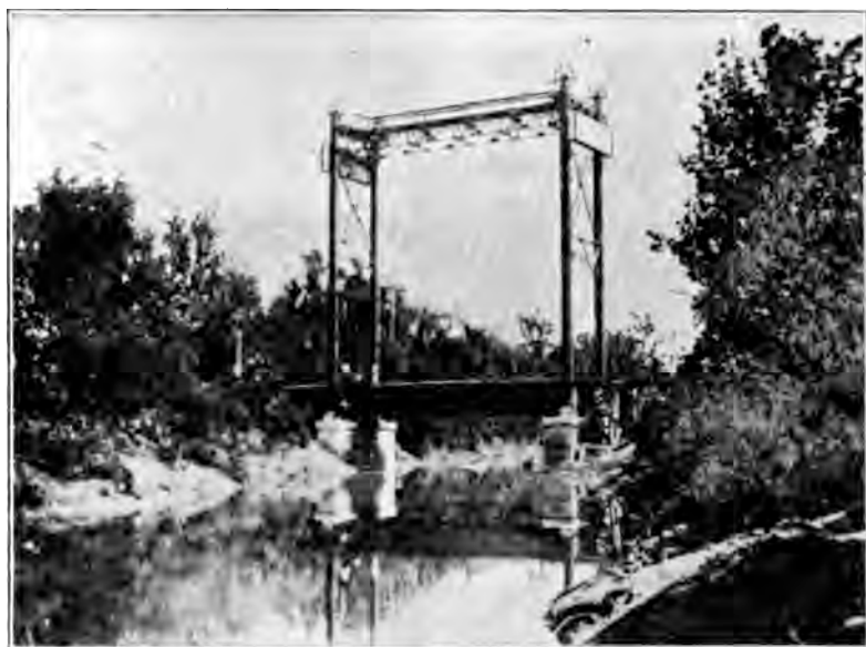
FIG. 31h. Vertical Lift Bridge over the Big Choctaw Bayou, Louisiana, on the Line of the M. L. and T. R. R. & S. S. Co.—Span Down.
