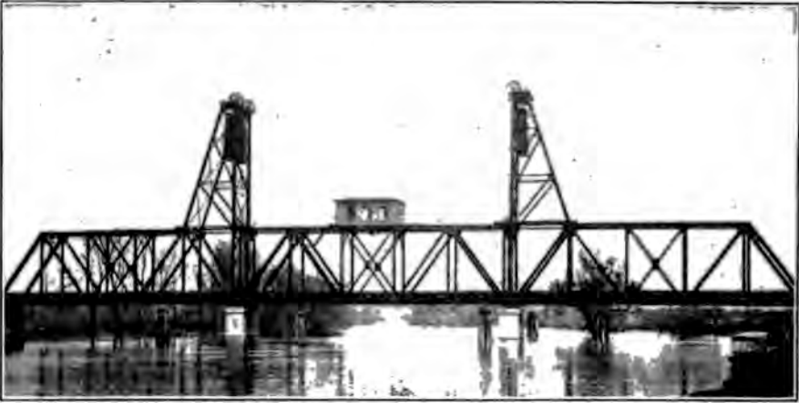
FIG. 31v. Louisiana & Arkansas Railway Bridge over Little River in Louisiana.—Lifting Span Down.
